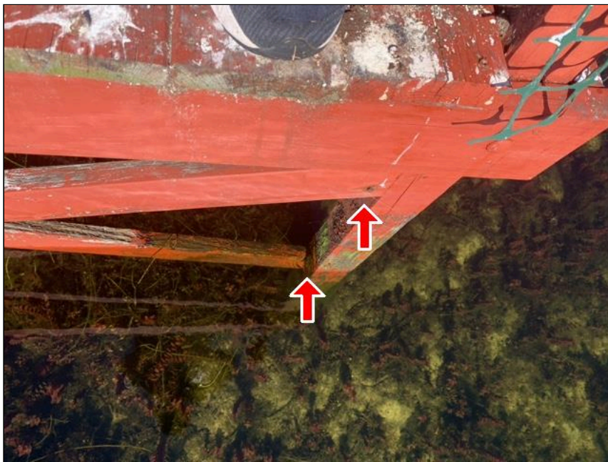
11.2 Item 11(Picture) not secured with fasteners here
