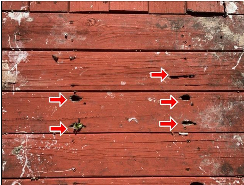
11.0 Item 2(Picture) large holes in boards where water entered fasteners
