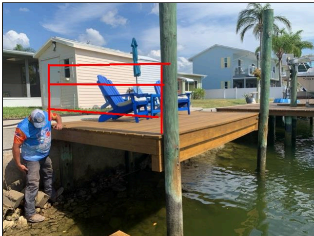
11.1 Item 1(Picture) no handrails present
