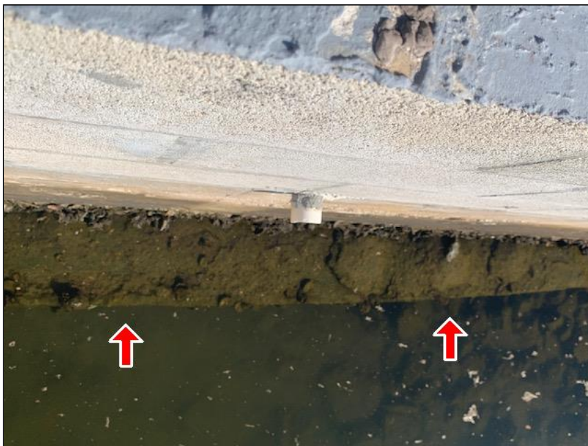
10.1 Item 1(Picture) footer undermined west corner out 15ft
