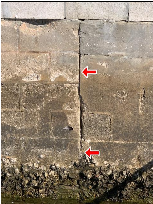
10.2 Item 1(Picture) cold joint crack
