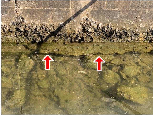
10.1 Item 2(Picture) washout visible under footer
