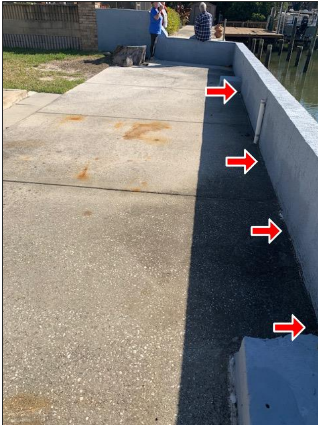
10.3 Item 1(Picture) drain holes blocked
